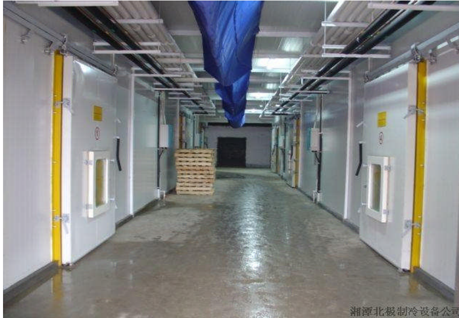
Figure 5: Medium-scale commercial CA storage facility in Hunan province
