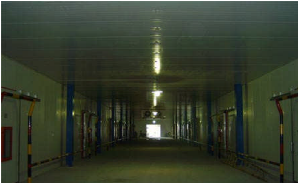
Figure 4: Large-scale commercial CA storage facility in Fujian province
